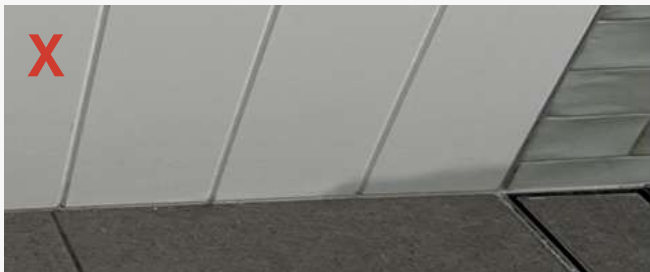
Panel used in a bathroom not installed on top of a skirting resulting in water wicking up the bottom of the panel and damaging it
